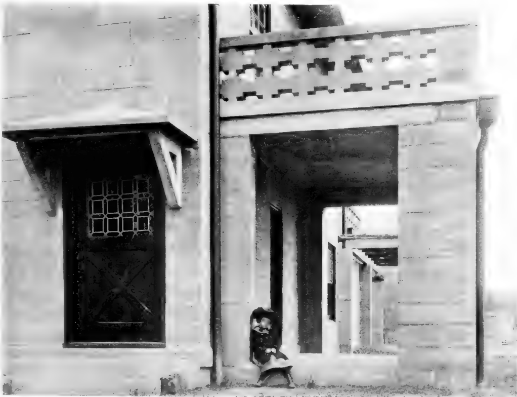
16—The Hood Over the Entrance-Way, and the Columns to the Porch are Made of Reinforced Concrete
